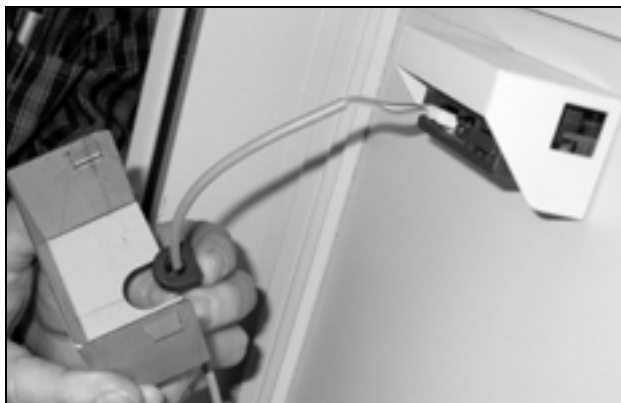
Fig. 16: Insert the cable sleeve
